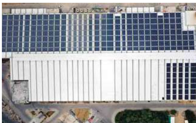
Expansion of Solar Power Plant up to 2.3MW
